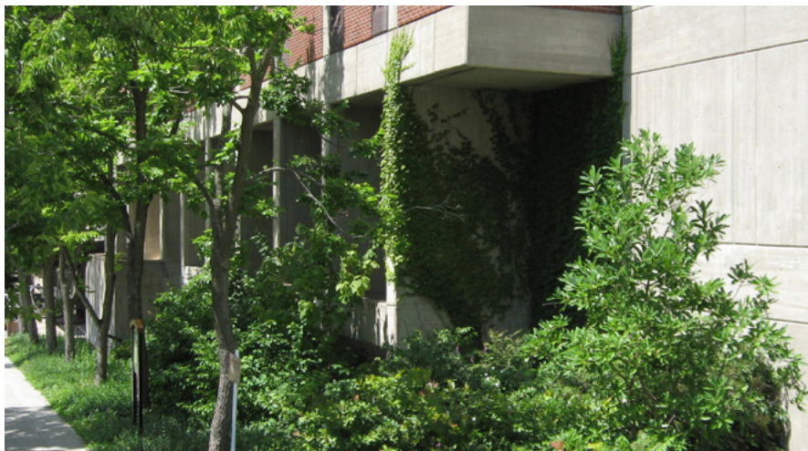
Rain garden (Photo: Wikimedia Commons)
